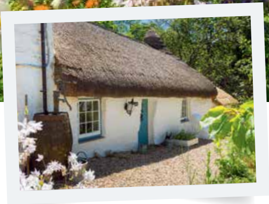
ABOVE The newly thatched roof is visible on the left LEFT In 1800, there were around one million thatched buildings; today there are just 24,000 listed buildings. The rise of the combine harvester abetted this decline – the straw it cuts is too short to be used in thatching
